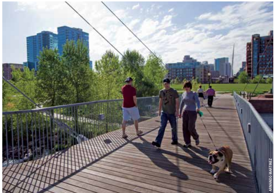
The Platte River Bridge, a pedestrian bridge over the South Platte River in Commons Park, is aligned with the Millennium Bridge and 16th Street in downtown Denver. This bridge, together with the Millennium Bridge and a third bridge over Interstate 25, has created a new and transformative nonvehicular commuting and recreational pathway within the city.
