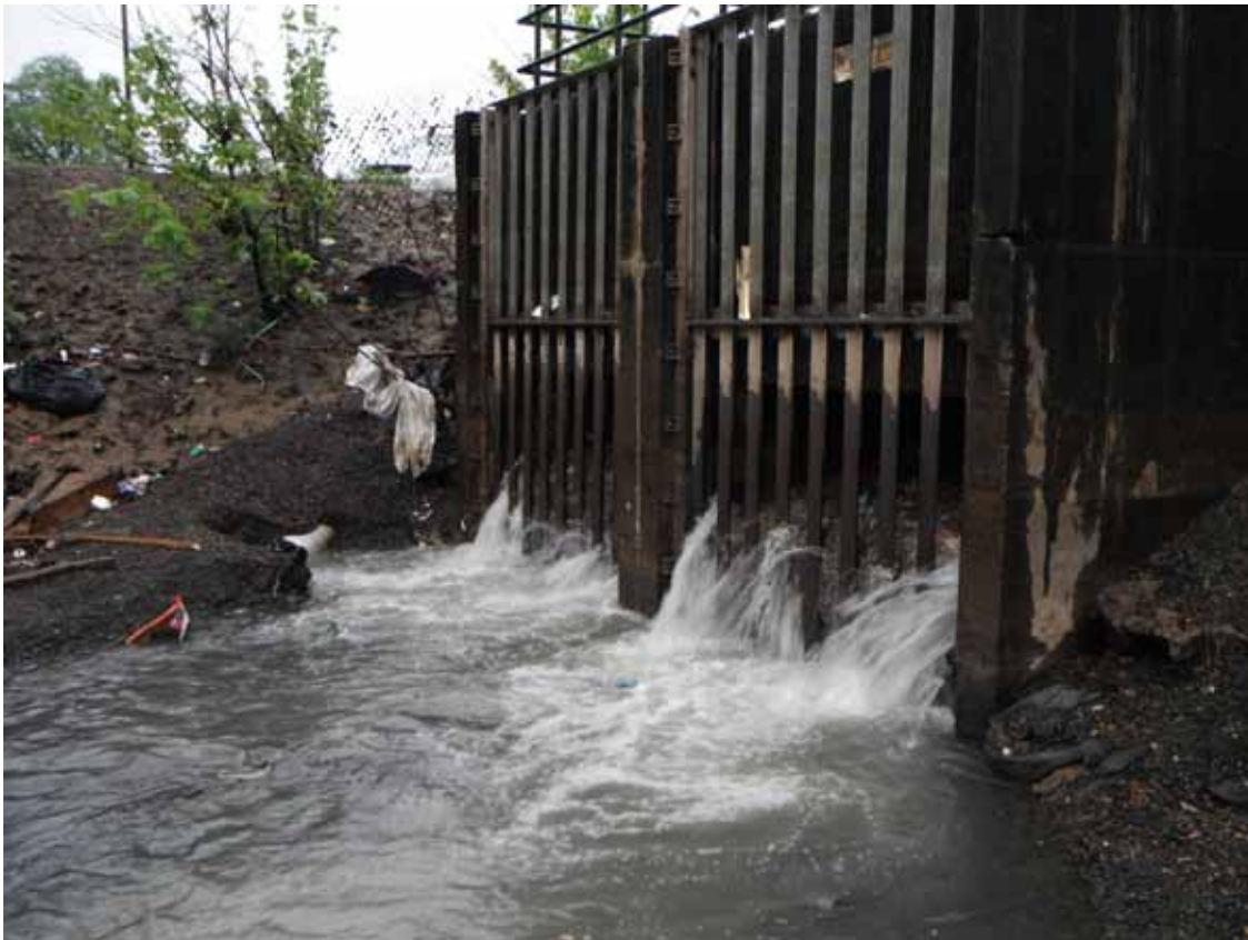
Figure 2. Combined sewer overflow (Photo courtesy of EPA)
