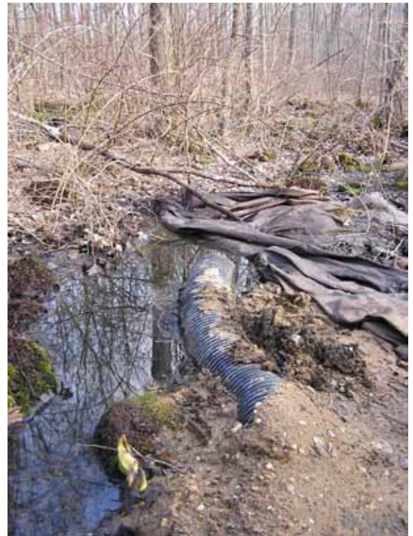
Figure 3. Illegal discharge of septic system effluent to a local waterway (Photo courtesy of EPA)
