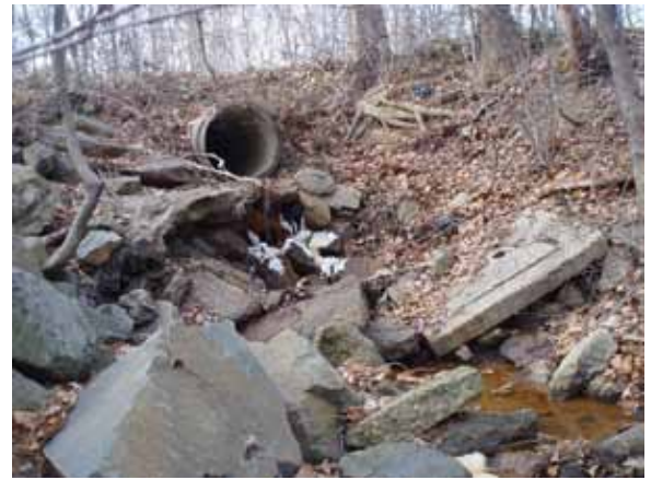
Figure 4: Visual Evidence of Sewage Debris
