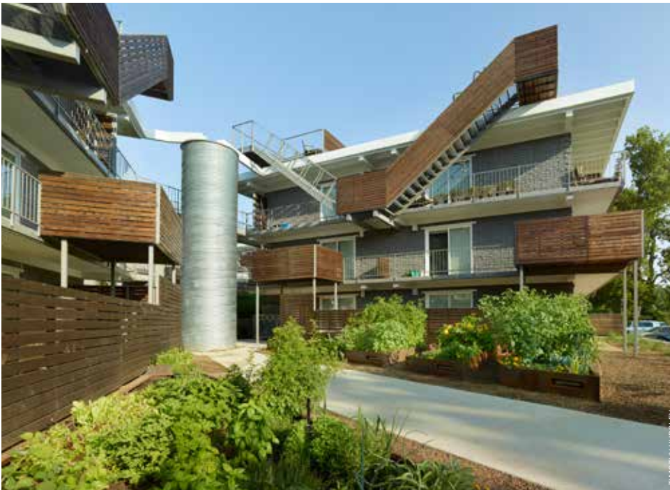
ECO Modern Flats offers a rental product that previously was unavailable to apartment dwellers in northwest Arkansas—urban, modern apartments with sustainable and healthy building features. The vertical cisterns for the development’s rainwater harvesting system, which were made from galvanized steel culvert pipes, serve as dramatic visual icons for the project.
