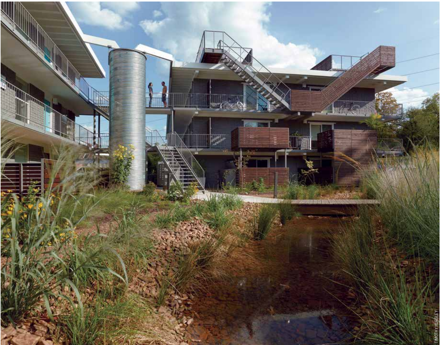
A courtyard rain garden, planted with native vegetation, diverts, slows, and filters stormwater runoff from parking areas.
