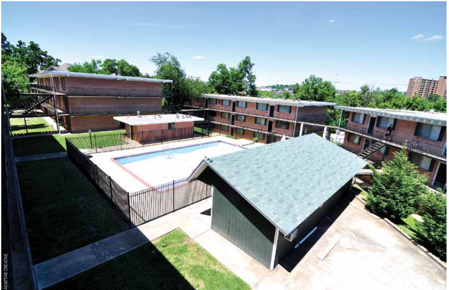
The buildings before renovation. The original four-building complex had great bones of precast concrete and split-face block.
