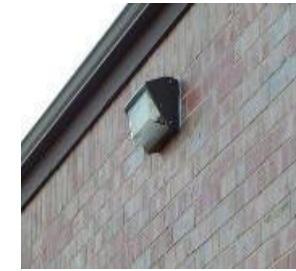
Exterior Lighting Retrofit
