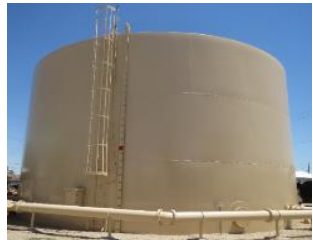
Water Distribution Controls
