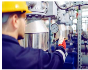
Combined Heat and Power Systems
