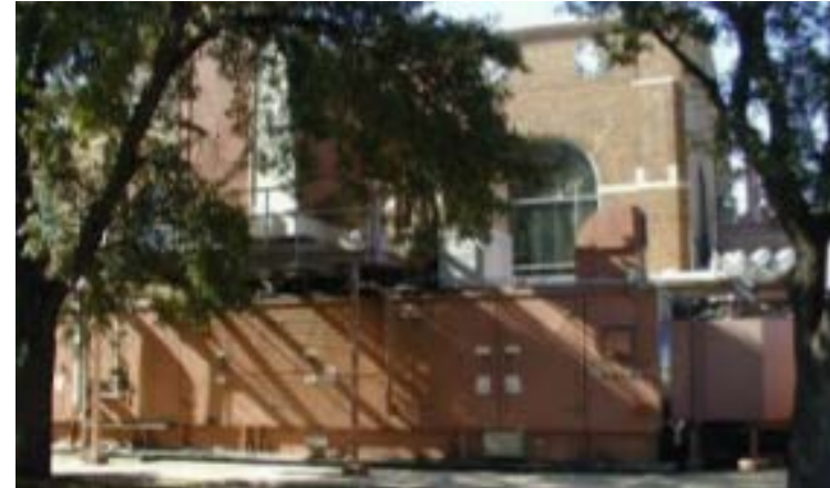
The Central Plant at Rice University houses the 7.4 MW CHP system, which produces 8,000 tons of chilled water and 130,000 lb/hr of steam
